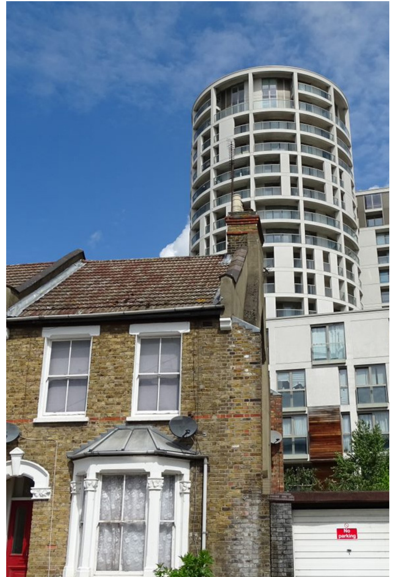
The white tower of Lantern's Court rises behind the Victorian terraces of Mellish Street. Such juxtapositions are typical of urban insertions.
