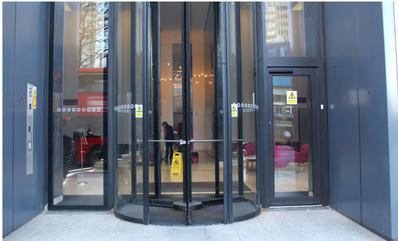
Entrance of Strata SE1, with cleaners visible inside.
