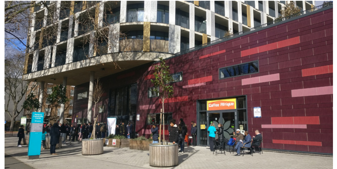
The ground floor of Pembury Circus caters to the diverse neighbourhood with a Peabody-run community centre, Coffee Afrique and (just to the right out of shot) Café Vincent, with 'all-day modern Euro eats & craft beers'.
