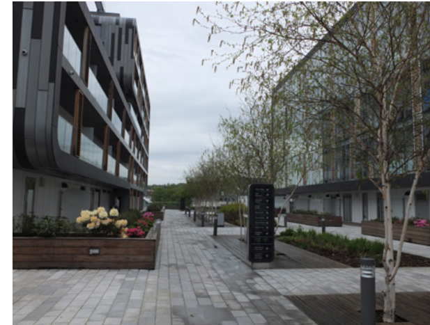
Woolwich Central, Woolwich
