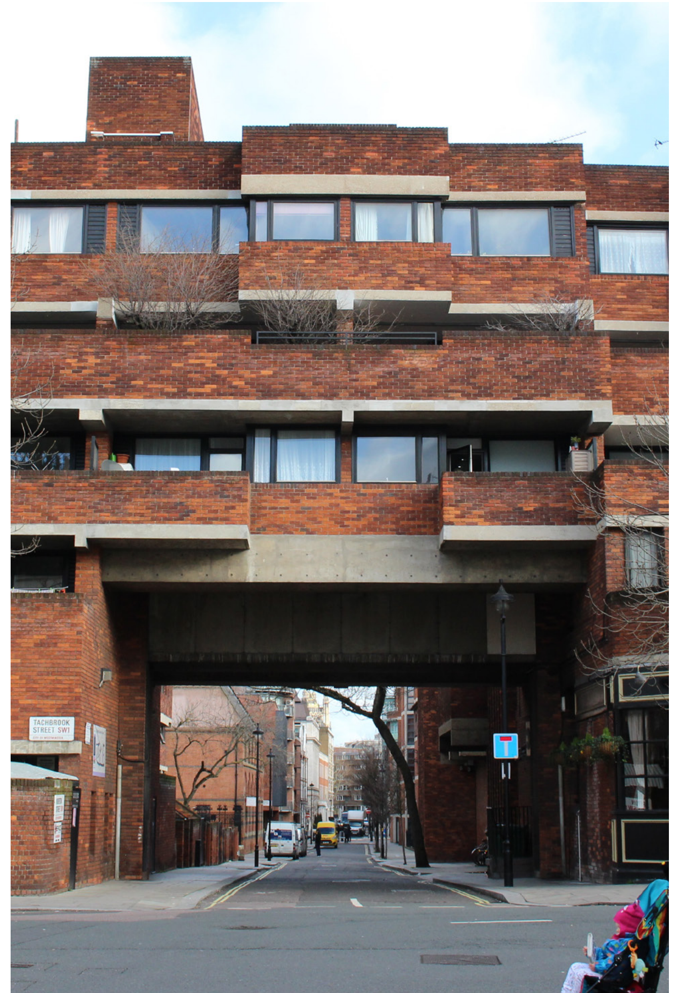
The buildings of Lillington Gardens straddle Moreton Street. This historic estate was considered dense when built in the 1960s.
