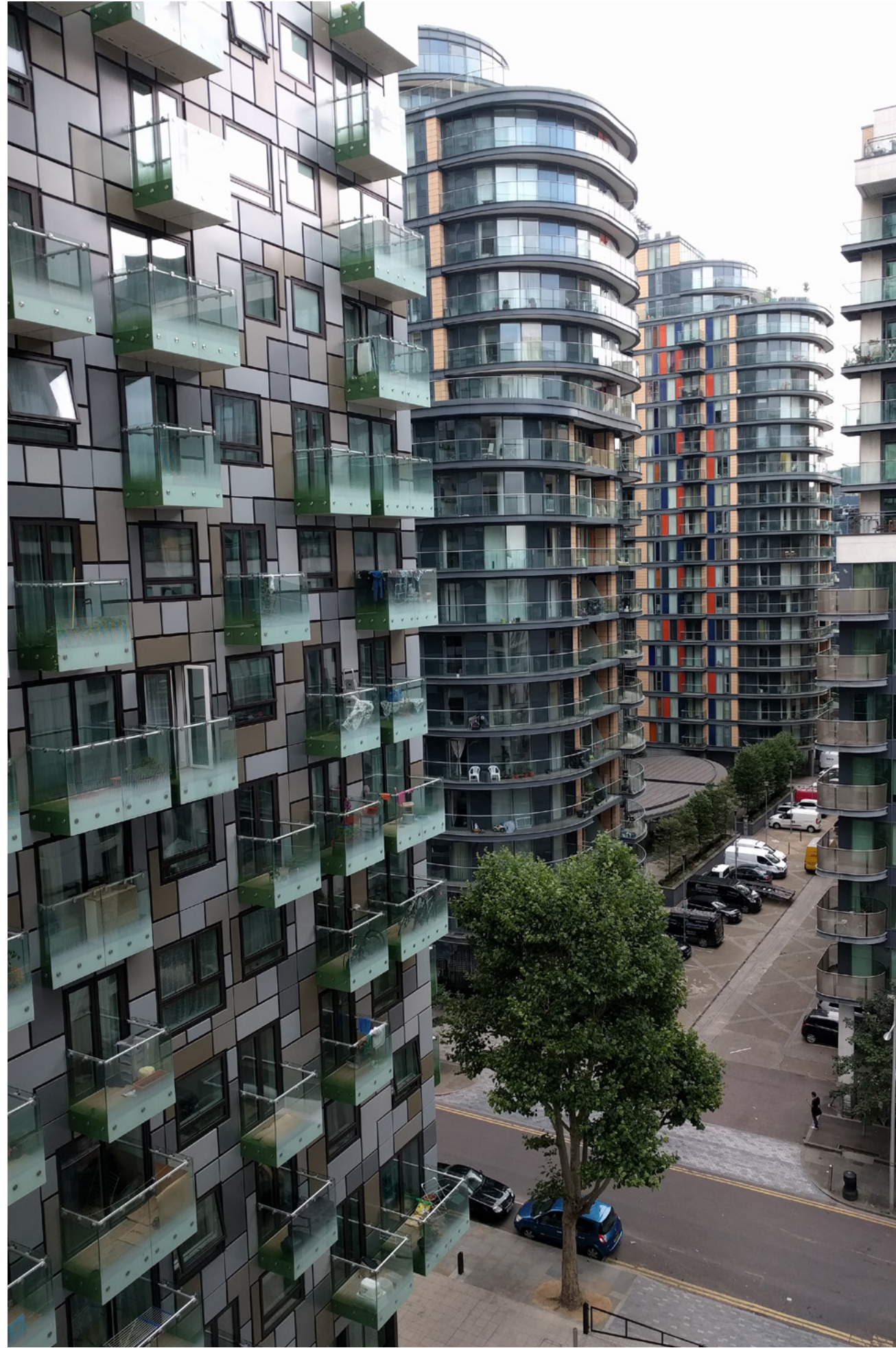
An emerging neighbourhood of high-density schemes on the Isle of Dogs, south of Canary Wharf. Floor-to-ceiling windows or entire glass walls are common as they admit more light to deep rooms.
