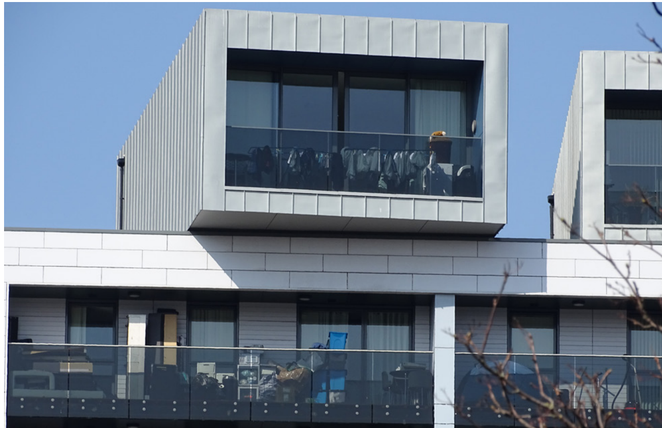
Upper floors of Thurston Point. Note the belongings stored on the balconies.
