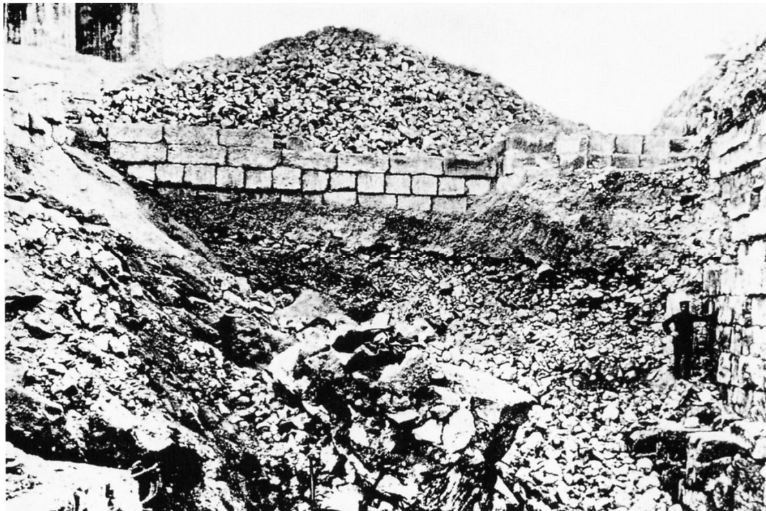
Fig. 08 Digging on the Acropolis (south of the Parthenon). c.1870
