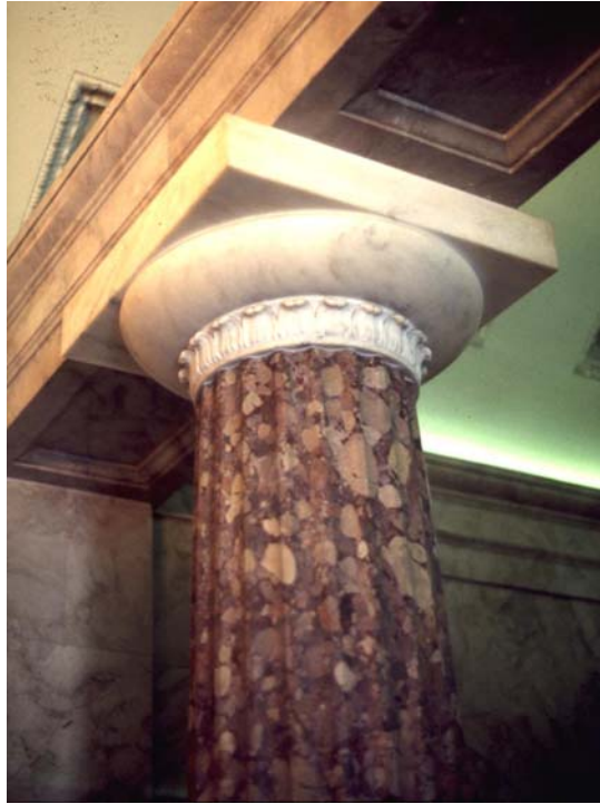
Fig. 15 Washington, DC. The Capitol. Greek Doric columns in the room under the Old Senate. Architect: Charles Bulfinch.
