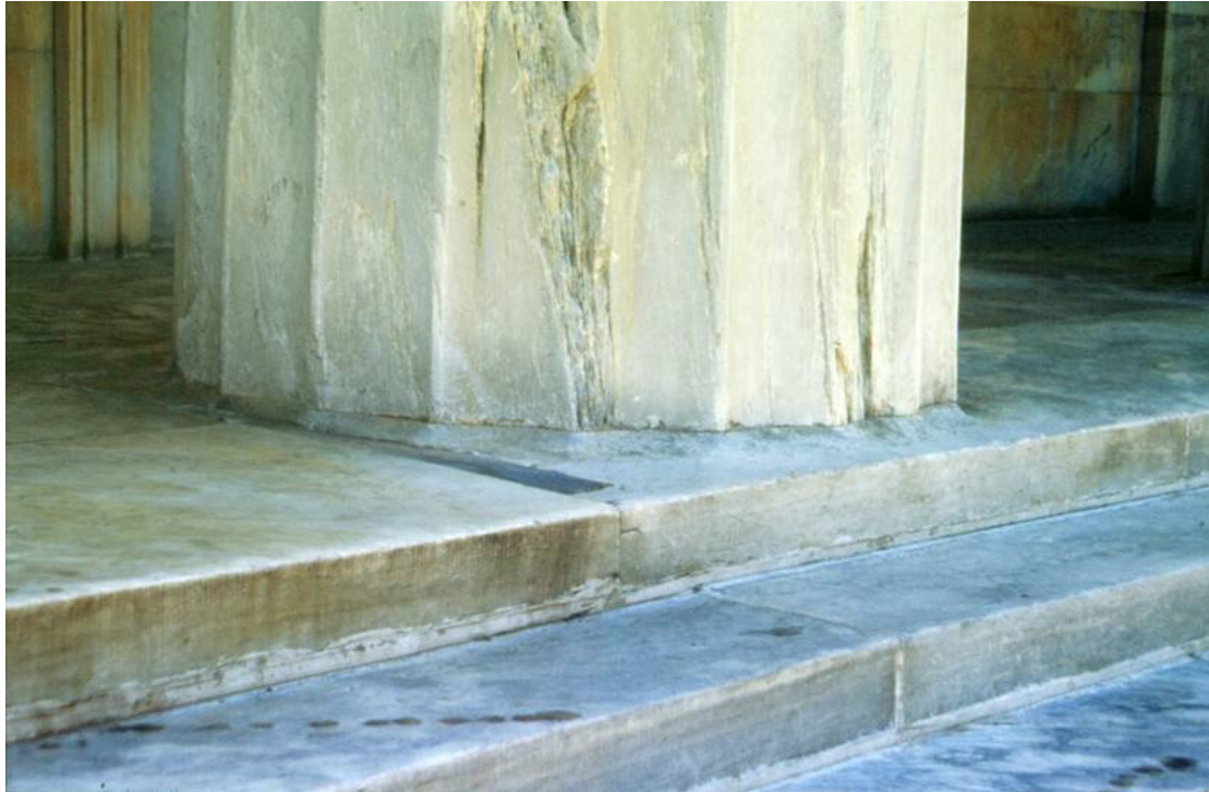
Fig. 22 Philadelphia, PA. Second Bank of the United States. Drum of marble column set on the floor as in antiquity.
