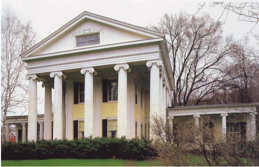
Fig. 29 Orwell, VT. Wilcock Cutts House. Architect: Thomas Dake. Alteration to present appearance 1843.
