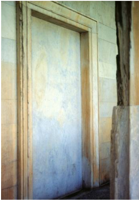
Fig. 37 Philadelphia, PA. Second Bank of the United States. 1819/24. Door, later filled with masonry.
