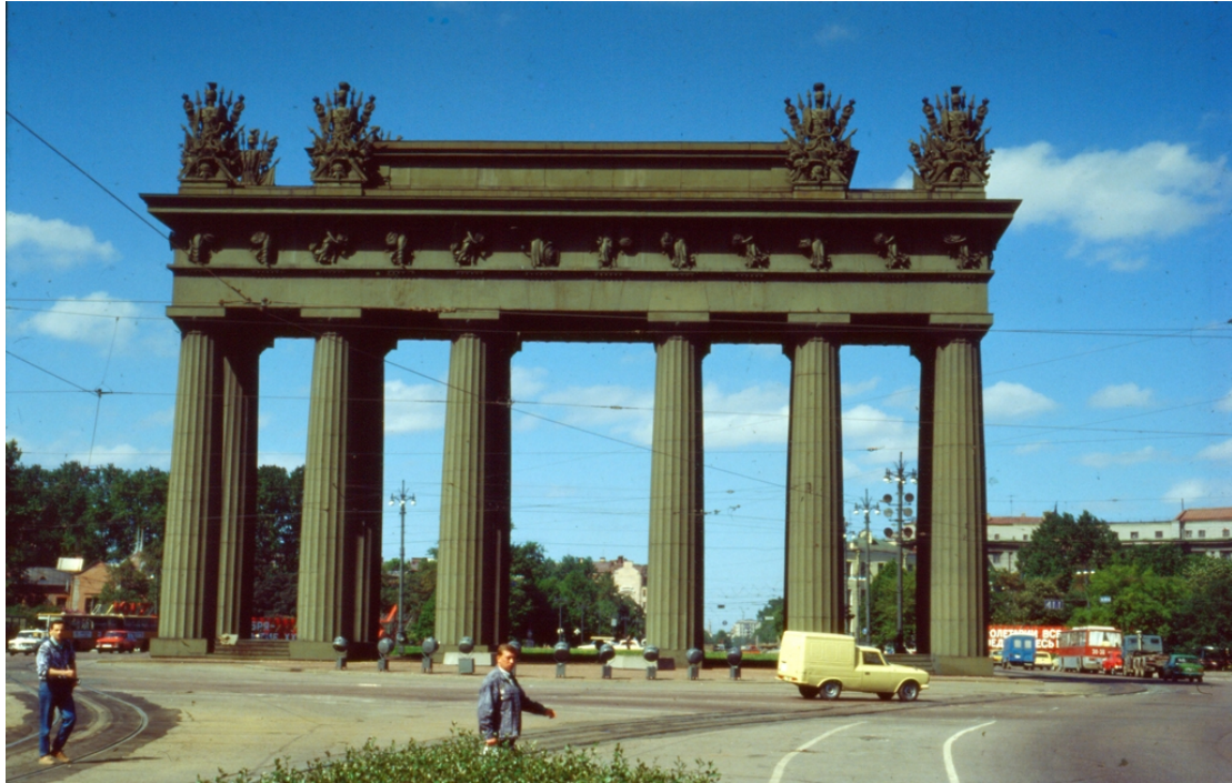
Fig. 11 "Moscow-Gate" in St.Petersburg. Architect: W.P. Stassow. 1838.
