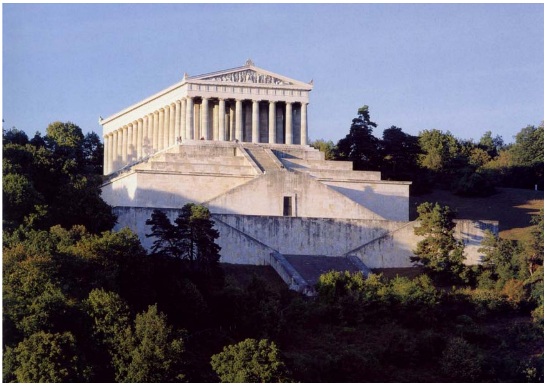
Fig. 10 Walhalla near Regensburg, Germany. Architect: Leo von Klenze. 1821/42.
