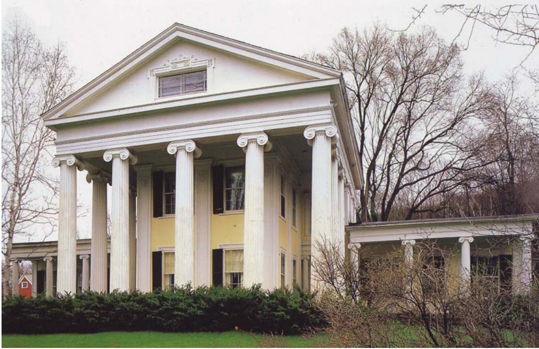
Fig. 29 Orwell, VT. Wilcock Cutts House. Architect: Thomas Dake. Alteration to present appearance 1843.
