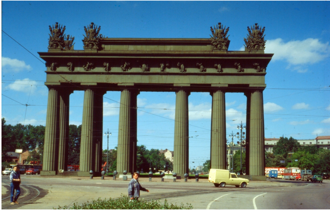
Fig. 11 "Moscow-Gate" in St.Petersburg. Architect: W.P. Stassow. 1838.
