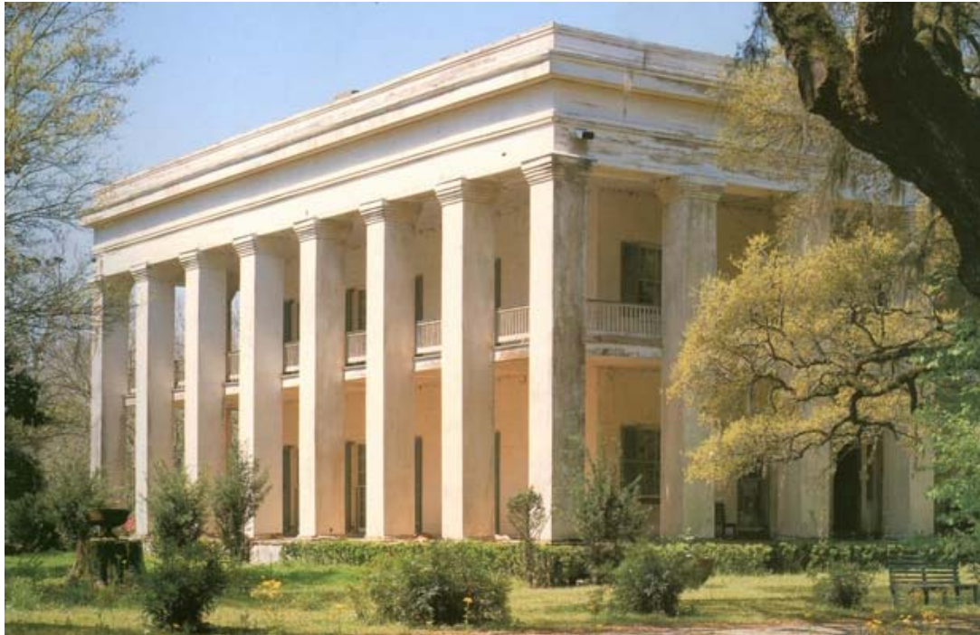
Fig. 39 Belle Helene near Napoleonville, LA. Architect: James Gallier. 1840/41.
