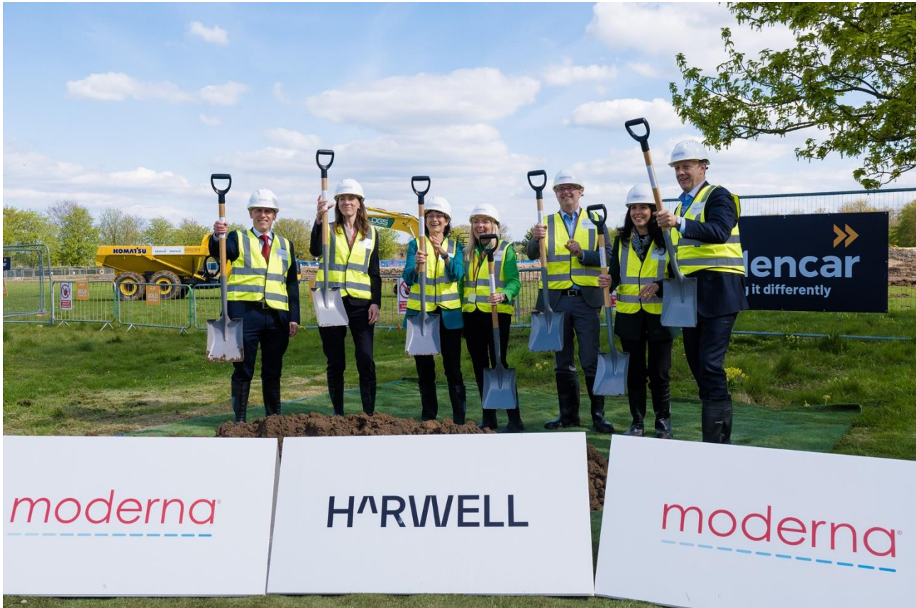
Figure 1: Launch of work on the Moderna Innovation & Technology Centre, Harwell, April 2023 (Credit: Tom Weller Photography)
